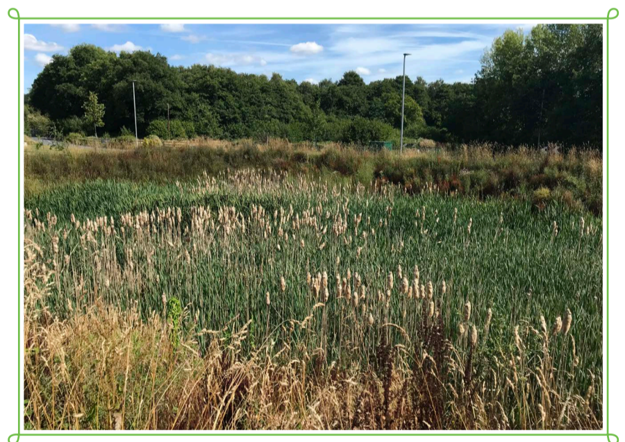
Example of a sustainable attenuation basin
