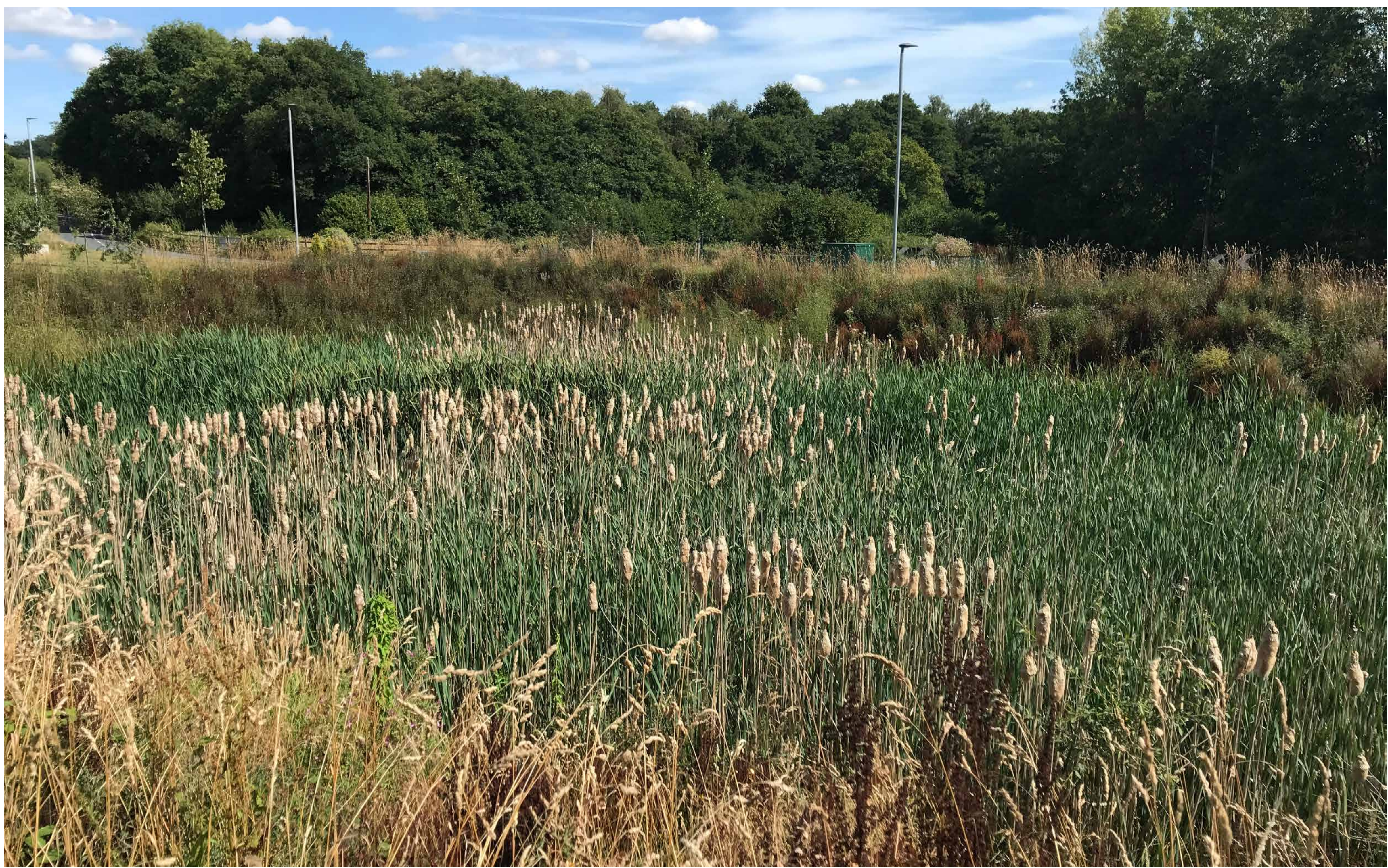
Example of a sustainable attenuation basin
