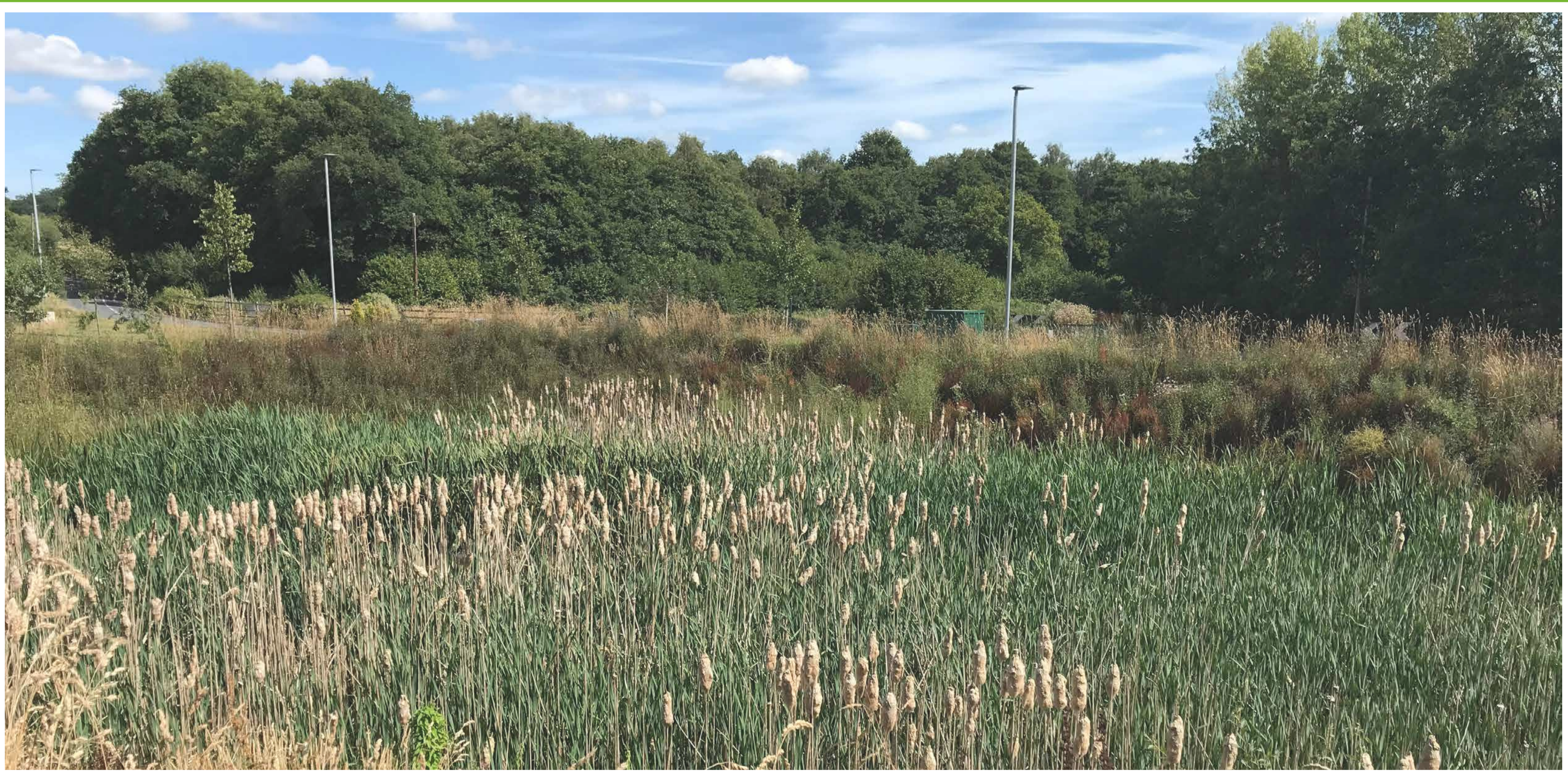
Example of a sustainable attenuation basin
